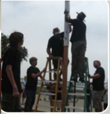
Installation of a Ventura, CA SLAP pole
